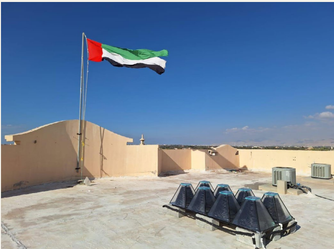
Figure 37: Flat-packable, self-assembled solar thermal collector installation in a household in Ras Al Khaimah
