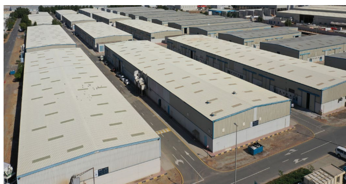
Figure 30: Al Ghail Industrial Zone, Ras Al Khaimah
