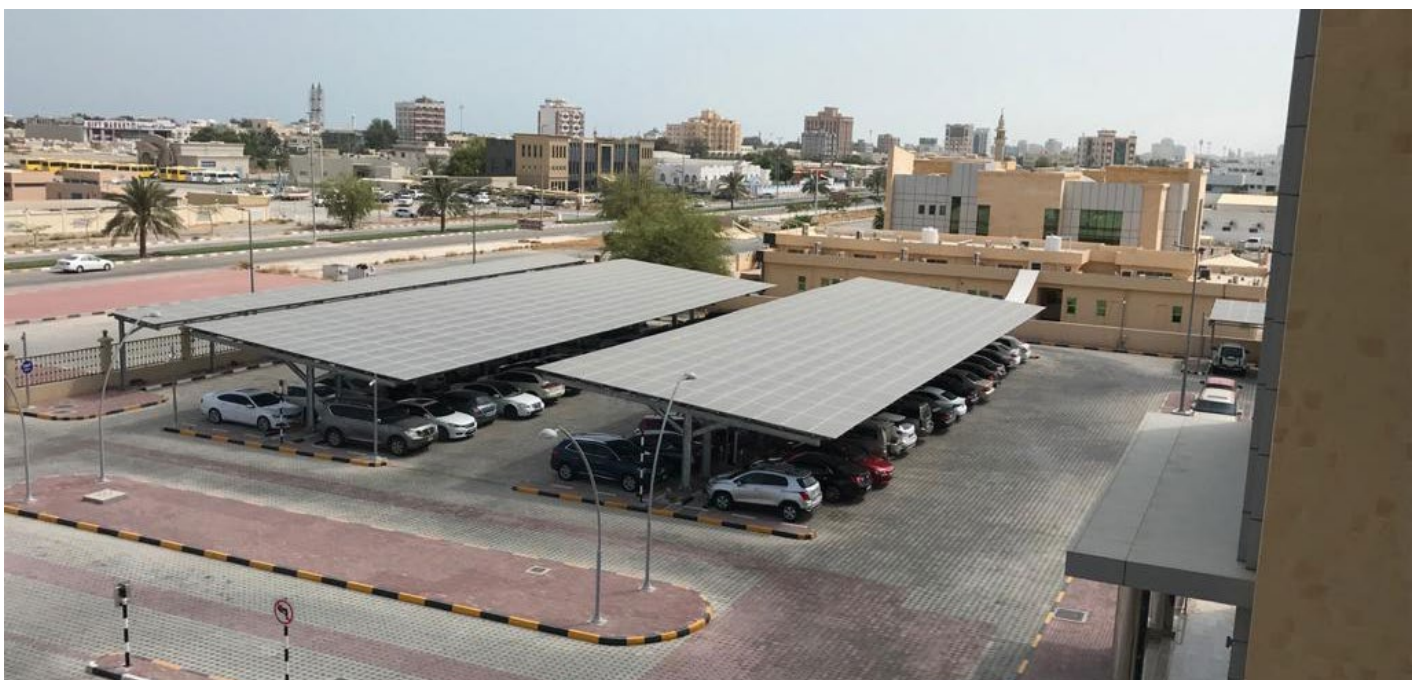
Figure 10: Solar carport at Ras Al Khaimah Municipality
