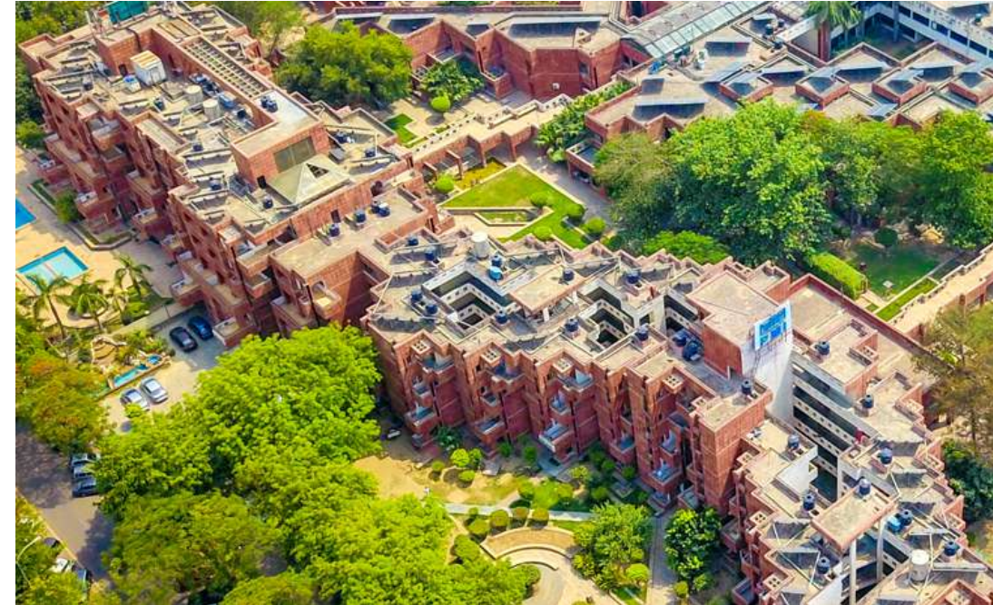
NTPC's Power Management Institute
