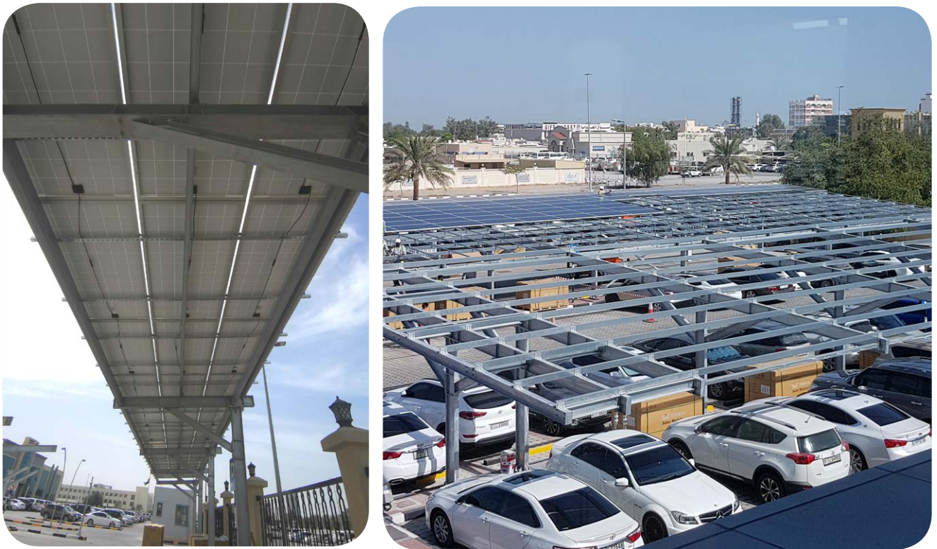
Figure 37: Construction of solar carports at Ras Al Khaimah Municipality
